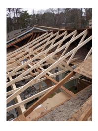
The damage to the roof was so severe that we needed to completely redo the framing and decking for the large section of the roof.
