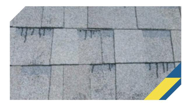
These stains and runs indicated to us that the shingles were defective and would need to be replaced to in order to ensure the longevity, value, and lifetime of the roof for the customer.
